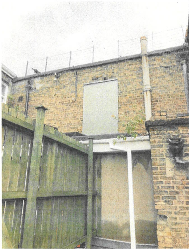
Above: My rear window covered with plywood (& subsequently painted!)
