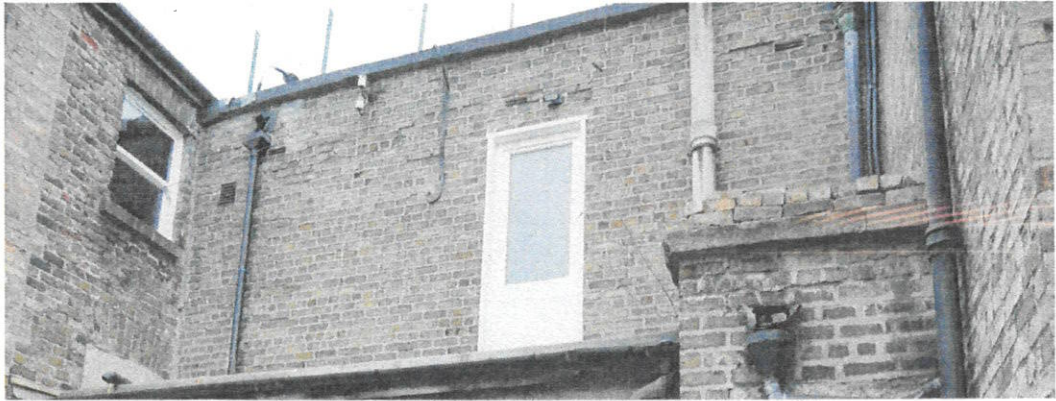
Above: My rear window before being blocked with plywood.
